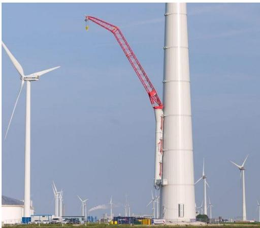
Figure 44: The Lagerwey climbing crane luffs its boom hydraulically, [source: [108]]
