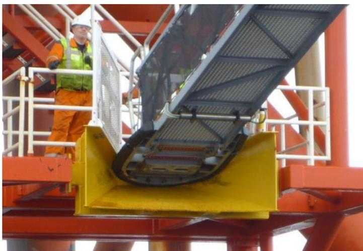
Figure 26: V-shaped landing zone for the motion compensated gangway, [source: [76] with permission by Ampelmann].
