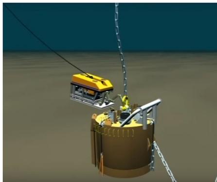
(a) A ROV pumps water out of the top suction port after sealing pile top valves. Pile top and ROV instrumentation contribute to a precise installation. [Source: <https://intermoor.com/press-releases/how-suction-piles-work/>].
