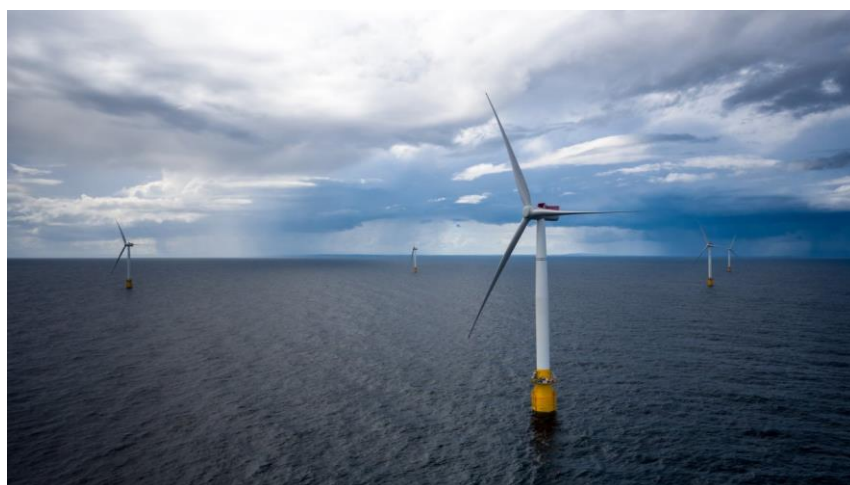
Figure 14: Hywind Scotland floating wind farm [Source: Equinor, Øyvind Gravås / Woldcam - Statoil ASA]
