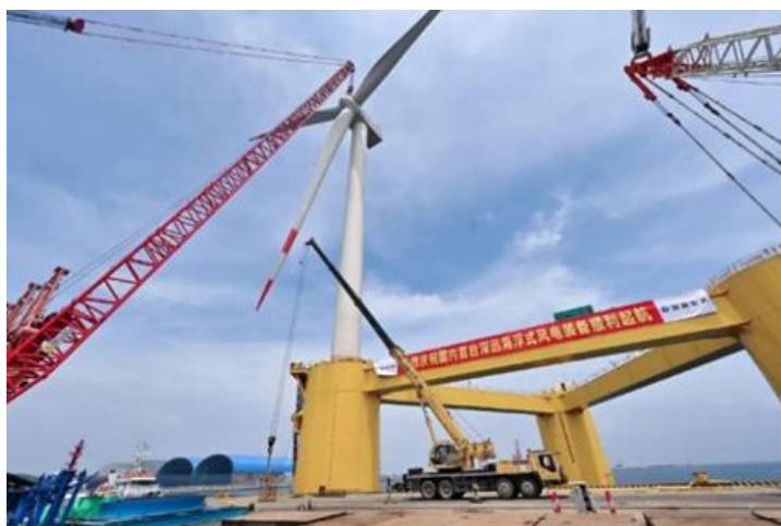
Figure 13: Fuyao semi-sub floater, equipped with a 6.2 MW typhoon-resistant wind turbine [Source: CSSC]
