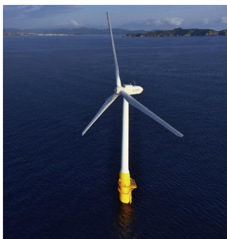
Figure 15: 2 MW FOWT on a hybrid spar foundation in Sakiyama, Japan [Source: Toda Corporation]
