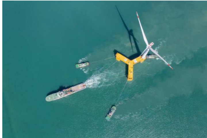
Figure 11: Sail-out of China’s first FOWT off the coast of Yangjiang City, July 2021 [Source: MingYang Smart Energy]
