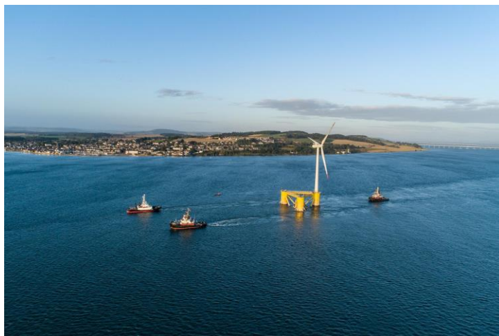
Figure 9: WindFloat semi-submersible floating foundation for Kincardine offshore wind farm [Source: COBRA Group]
