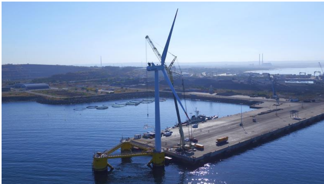
Figure 35: WindFloat at Sines quay side, while the turbine is being decommissioned, [source: [101]].
