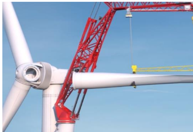
Figure 45: Blade installation at nacelle using the Lagerwey climbing crane, [source: [109]]
