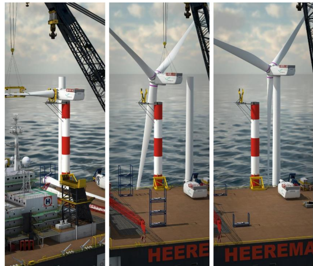
Figure 47: Visualization of RNA Assembly Process [source: with courtesy of HEEREMA, [111]]
