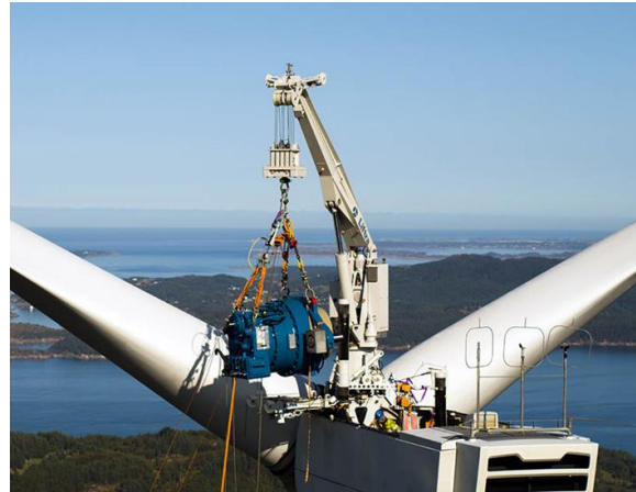
Figure 41: Self-hoisting crane changing gearboxes in a Nordex 2.5MW turbine, [source: [107]].
