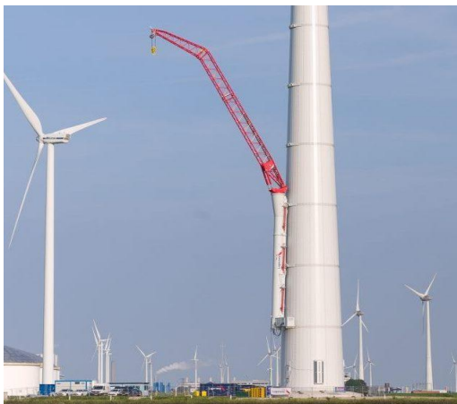
Figure 44: The Lagerwey climbing crane luffs its boom hydraulically, [source: [108]]
