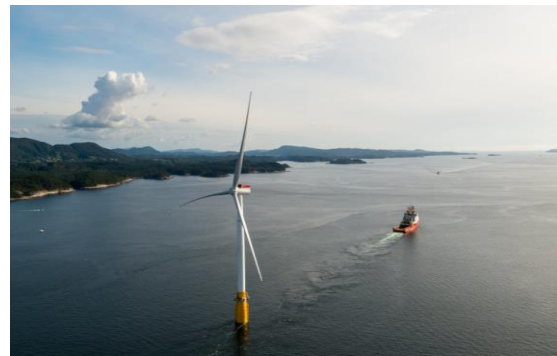
Figure 39: Turbine being towed to open waters, [source: [104]].
