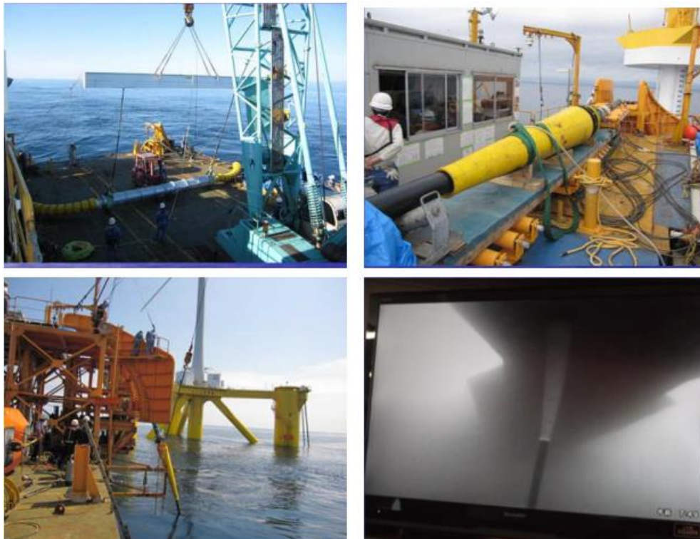
Figure 5.1-10 – Pictures from the Installation Procedure of Fukushima Demonstrator Project; Source: [15]
