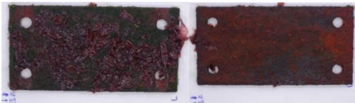
Figure 9- 3: Bare steel at Tidal area. Face A (left) and Face B (right) [23]
