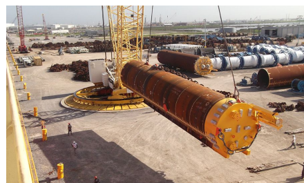
(d) A suction pile is being lifted at a fabrication yard. The mooring chain connection pad-eye is visible. Pad-eye is generally designed for loads inline with the mainplate. Some side loads are tolerable, but not full mooring loads. [Source: http://www.firstsubsea.com/products/smc/image-gallery.html ].
