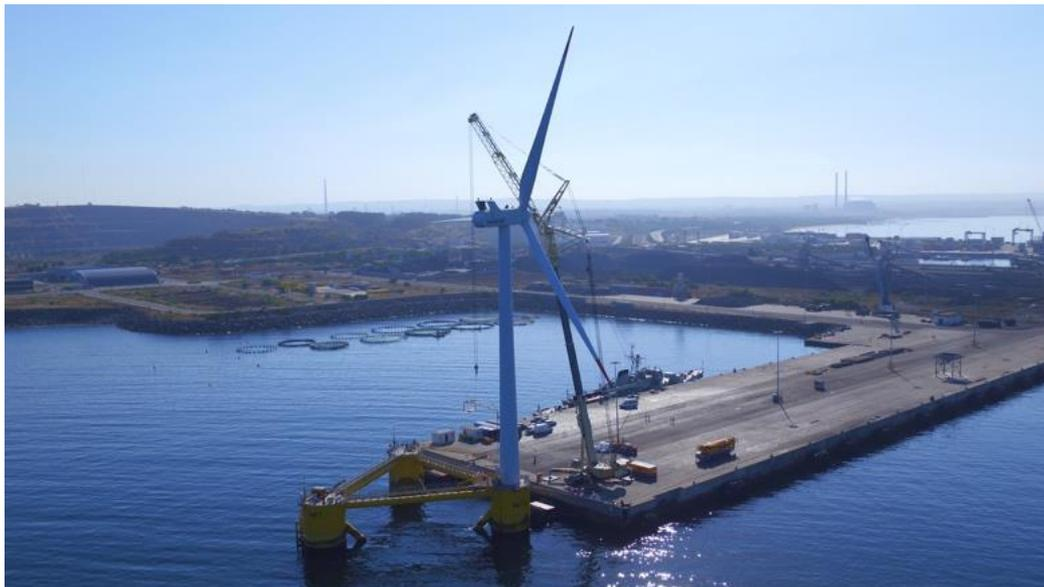
Figure 35: WindFloat at Sines quay side, while the turbine is being decommissioned, [source: [101]].
